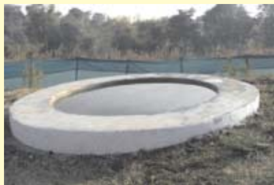
Water storage tank in nursery
